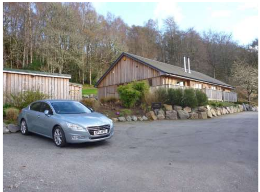
Weir Cottage is one half of the building on the right
