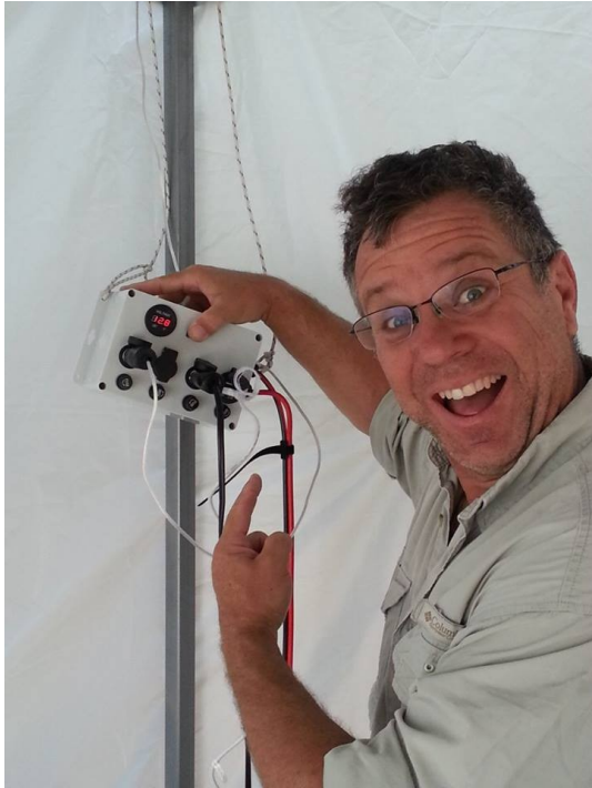
Ray seems well pleased with his power distribution box.
