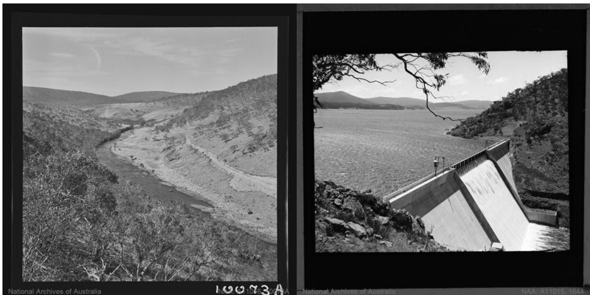
Before and after the construction of Tangtangara dam.
